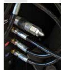
Nitrogen pressure test
