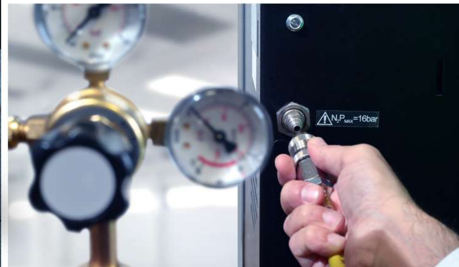
Nitrogen pressure control
